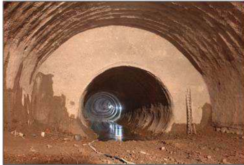
View of the cavern (and running tunnel) some days prior to collapse. The last eight lattice girders, beyond a fault in the foreground, did not fail (Nick Barton).
