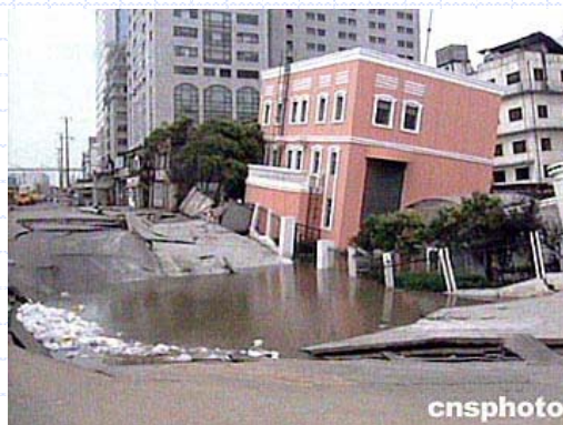
Colapso do Metro de Shanghai, China, 2003
