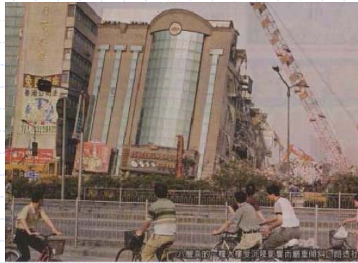
Colapso no Metro de Shanghai, China, 2003
