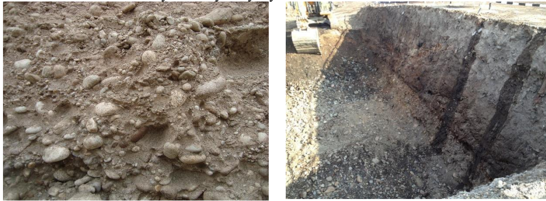
Figure 2. Details of the conglomerate found in the excavation area.
