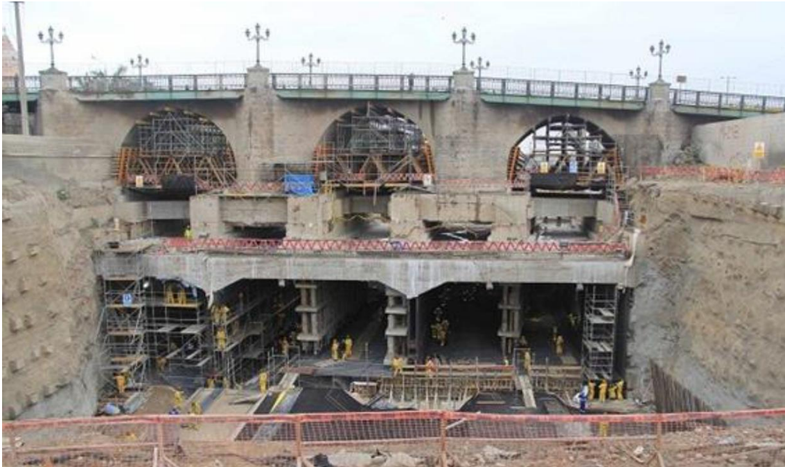
Figure 6. Tunnel construction beneath the historic stone bridge.
