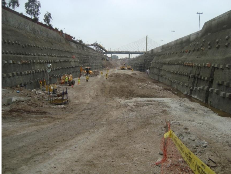
Figure 4. View of the slope excavation along the construction site.
